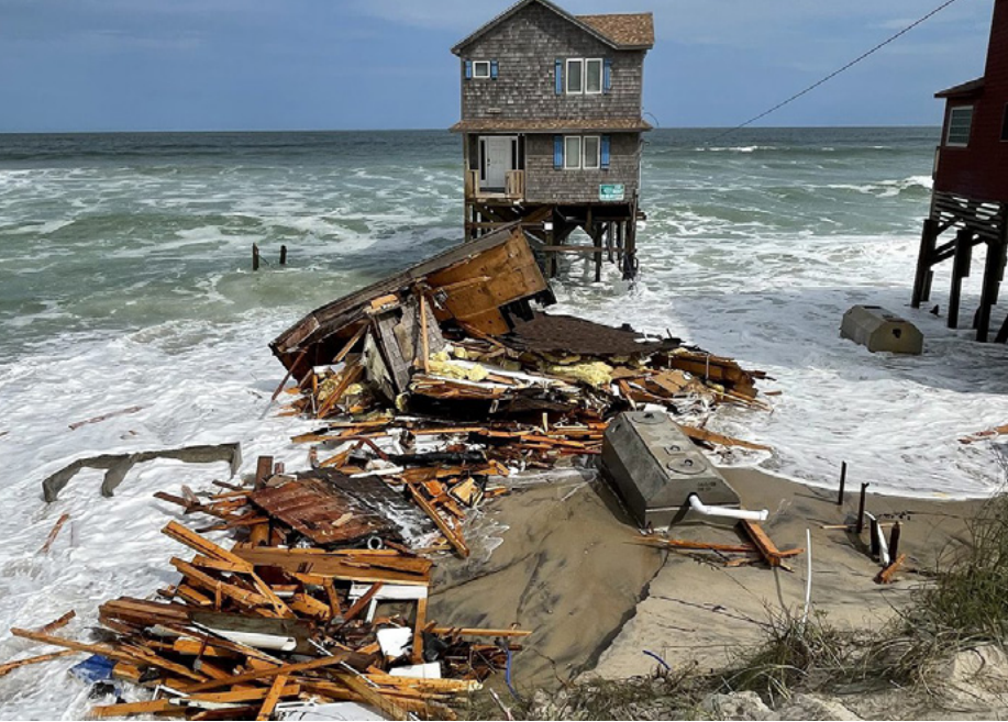
Adaptation to climate change may involve losing some human-made structures to sea level rise and storms. These seaside houses in the Outer Banks of North Carolina have been ravaged by the encroaching shoreline and erosion. (Image by National Park Service)
